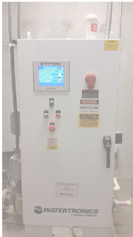
PUMP CONTROL PANEL
