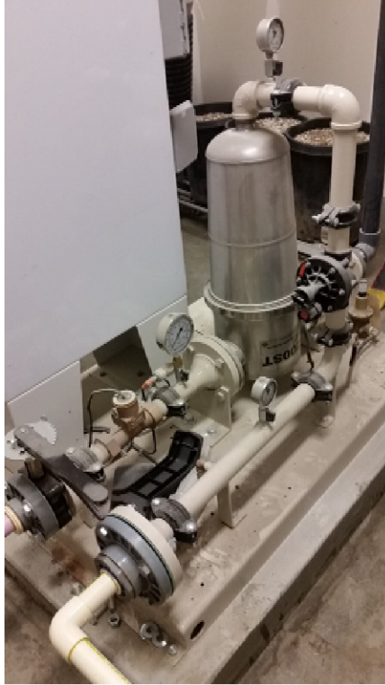
FILTER UNIT INSIDE STORAGE ROOM
