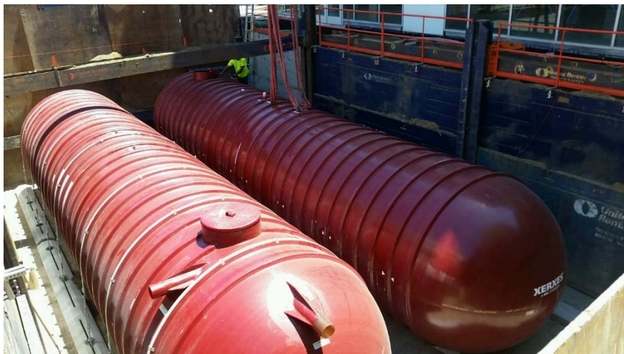
RAINWATER CATCHMENT SYSTEM INSTALLATION
